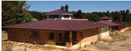
Members of the Pinoleville Pomo Nation built modern, wood-framed homes in Ukiah, CA. The breathable walls—consisting of straw bales and adobe-like cob, covered with a finish layer of clay-based plaster—prevent the buildup of moisture and mold. The rounded walls are in keeping with traditional Pomo architecture.<sup>3</sup>
